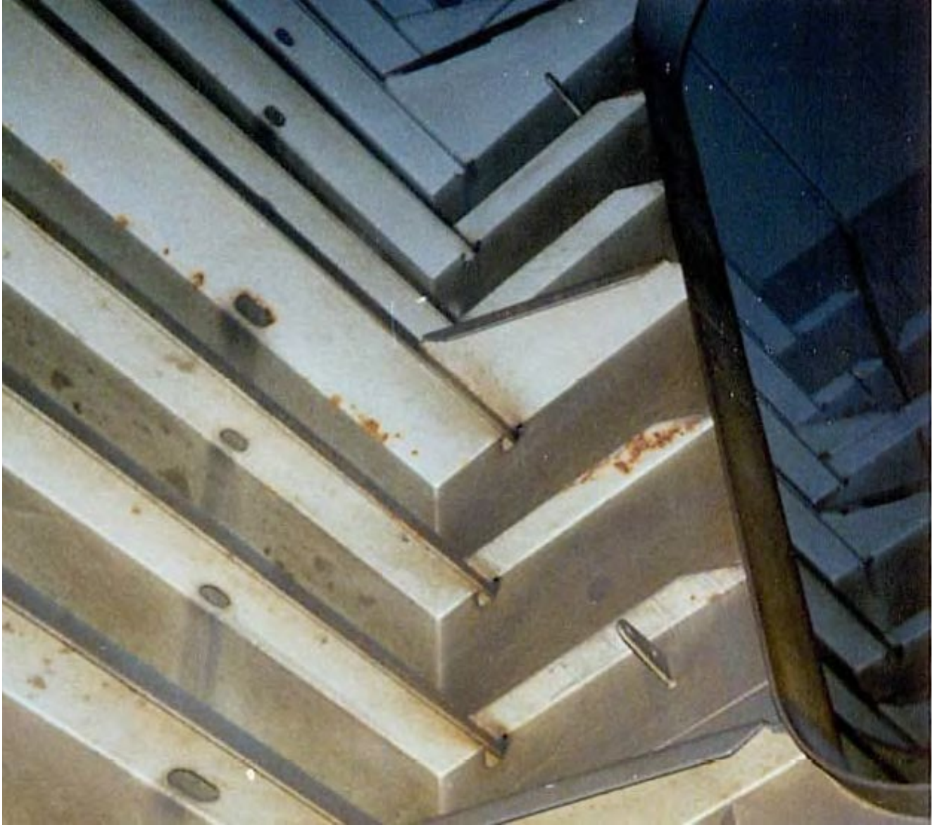
Good Coating Condition
